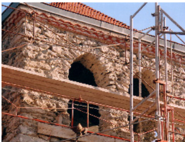
CHANTIER ECOLE SWEZZA
