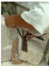
PHOTOS: CHANTIER ECOLE SWEZZA
